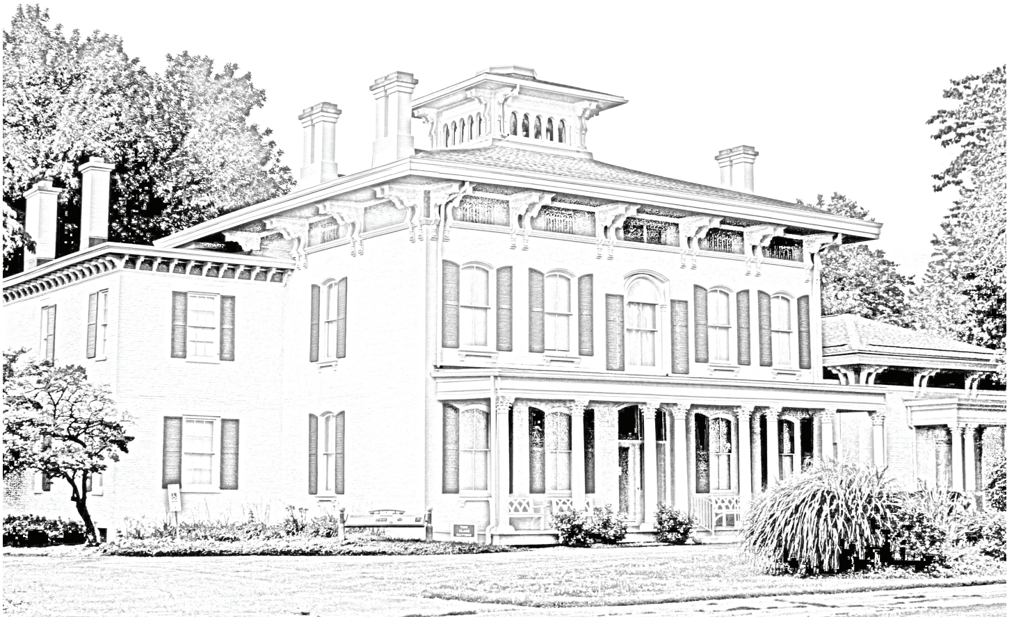
Edwards Place Historic Home, 700 N. Fourth Street, Springfield, Illinois www.edwardsplace.org
